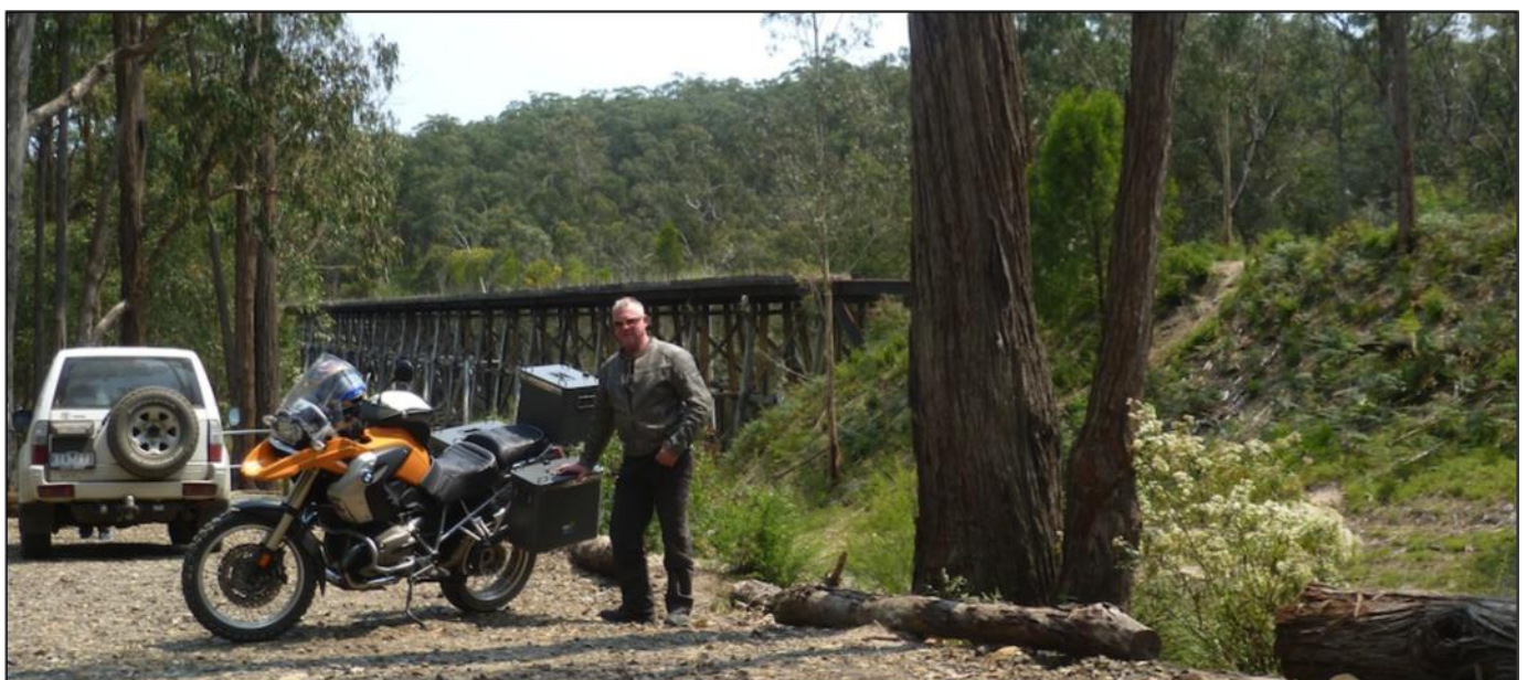
Figure 1 Historic wooden trestle bridge, Nowa Nowa, Vic
