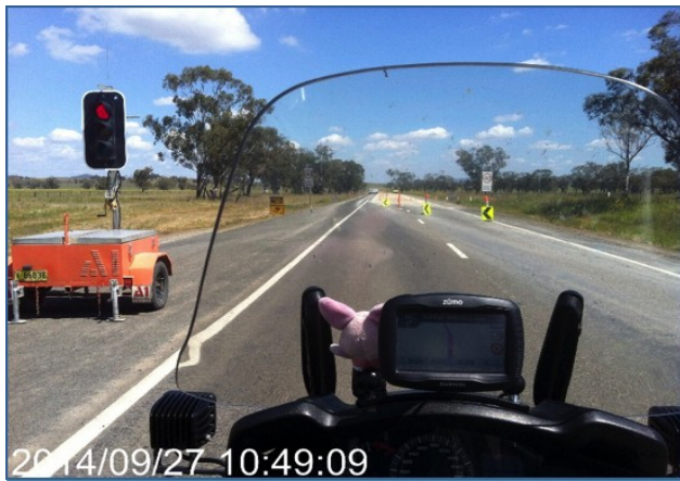
Roadwork's west of Tamworth
