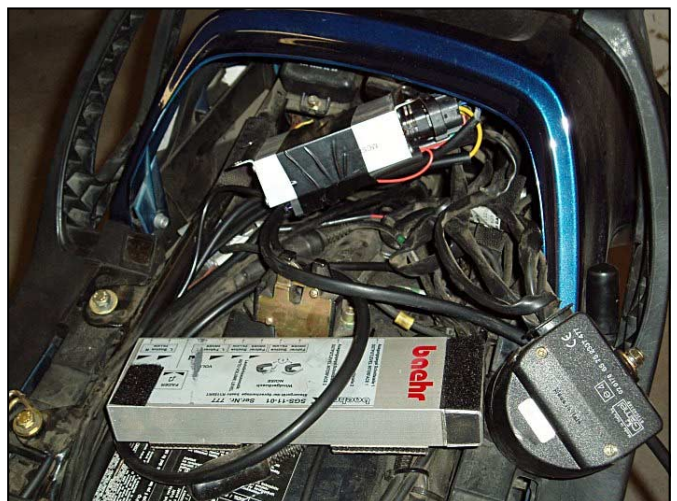
Shot of the ducktail during installation. Baehr unit out of position, cruise computer in the background and the semi-circular black thing is part of the alarm unit out of position to get at the nuts holding the rear light assembly.
